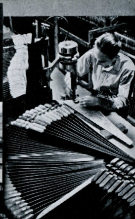
Placing handles on blades and tightening screws.
