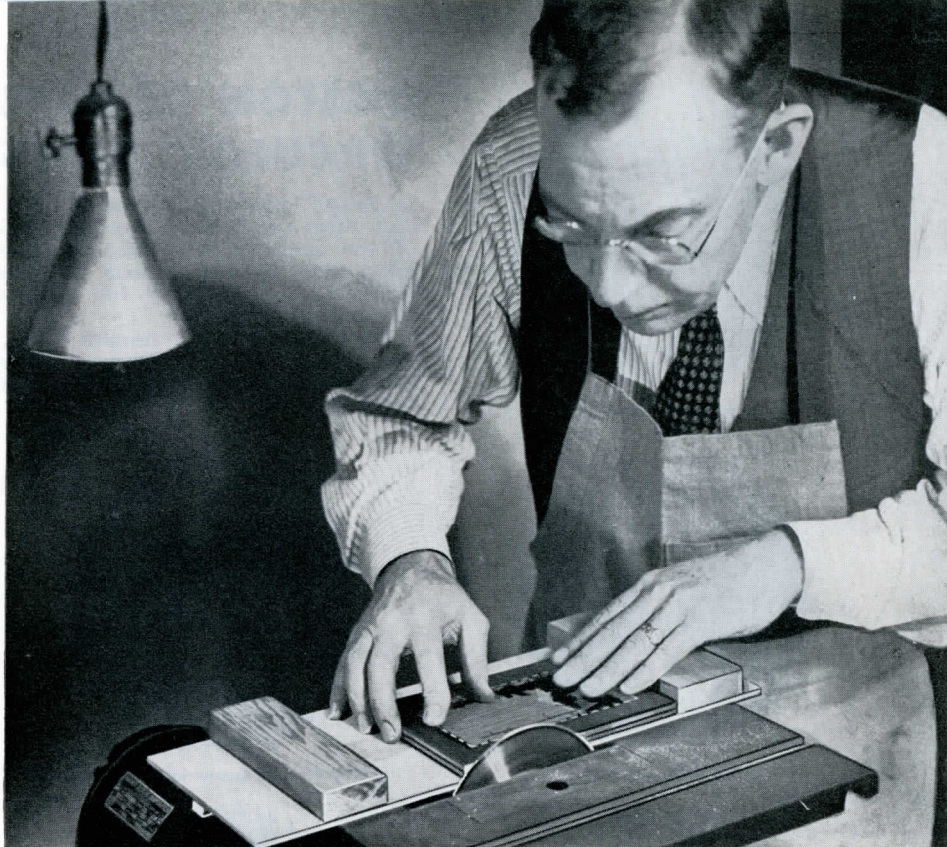
ABOVE —Trimming inlay picture with "square board" made of plywood with a strip to fit table slot tacked to bottom.
